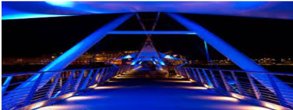
On Oct. 18, 2011, the new Tempe Town Lake Pedestrian Bridge opened, connecting the north and south shores of Tempe Town Lake. The bridge consists of 4 spans, each measuring 228 feet, weighing 165,000 lbs. The bridge protects the bladders of the dam from the sun and contains a built-in sprinkler system to cool the bladders when needed.
